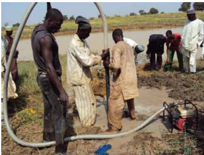
FIGURE 3.3: Washbore drilling
