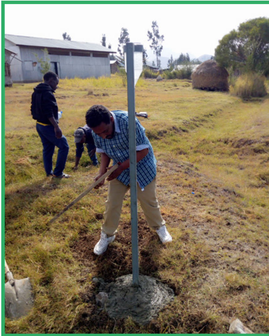
COMMUNITY RELAYS AND LOCAL PROJECT COORDINATOR INSTALLING GROUND WATER GAUGE
