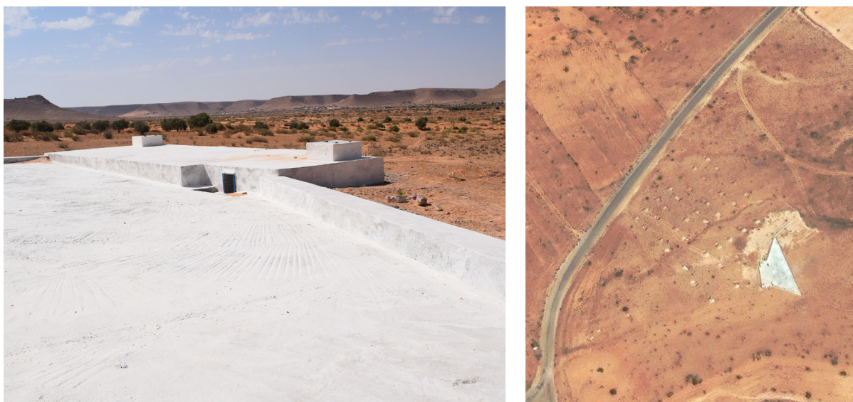
Photos of a water cistern being built by the project in the municipality of Beni Khedache, taken on location (left, © PRODEFIL) and by satellite (right, © Maxar Technologies)
