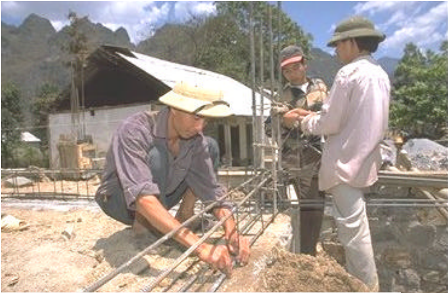
Ha Giang Development Project for Ethnic Minorities Construction workers build the project-funded district health centre in Yen Minh
