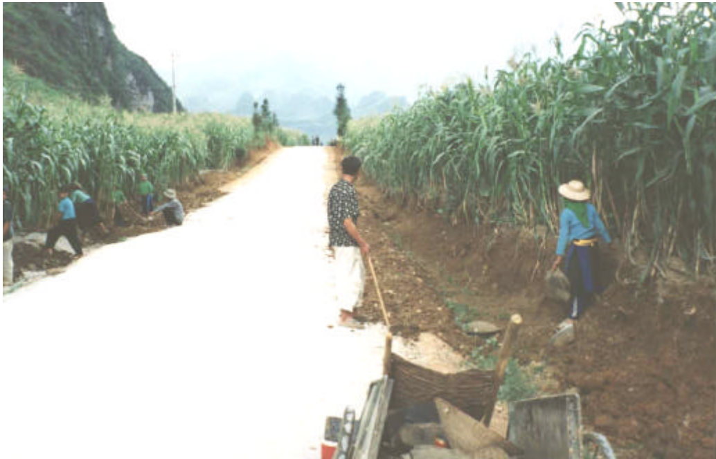
Agriculture Resources Conservation and Development Project in Quang Binh Province Rehabilitation of rural road.
