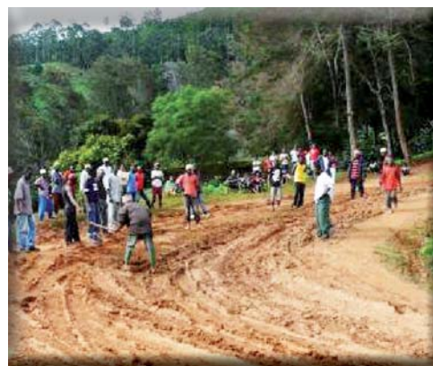
Access to markets - road upgrade and maintenance, Lushoto
