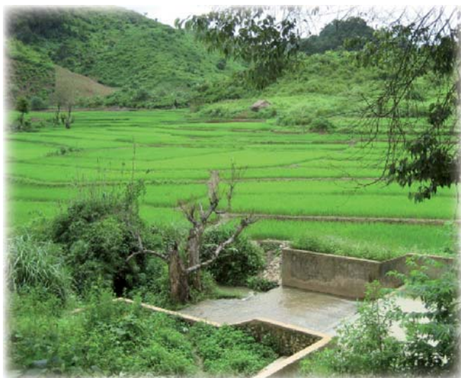
An irrigation weir constructed by the project in Nam Heng Neua, Xay district.
